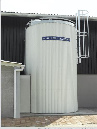
The silo is coated in a weather proof aluminium jacket in a 'off-white' colour.
