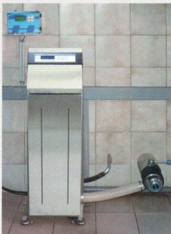
MIII control unit and outlet in the dairy.
